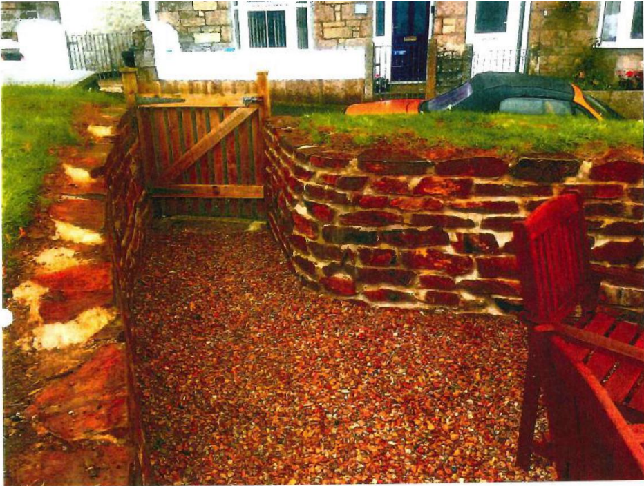
FIGURE 4: THE LAND AFTER THE MAY 2017 WORKS (LOOKING BACK TOWARDS 7 HARBOUR VIEW)
