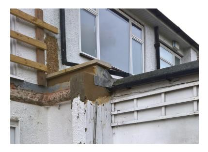
In this case I was the building owner's surveyor. This case involved the cutting away of a reinforced concrete balcony from a party wall. The Building Owner's builder did not follow the agreed method of cutting the balcony away from the party wall. The unauthorised use of a Kango in the removal of the balcony from the party wall, together with vibration caused cracks in the party wall in the Adjoining Owner's living room.
